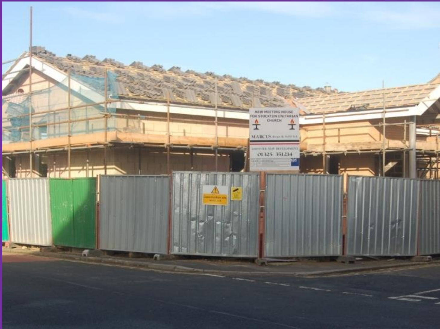
October 2006 The new building takes shape
